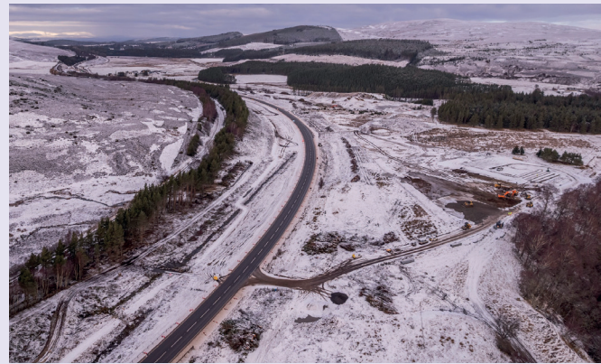
Image: Aerial view of the site compound under construction at Invereen
