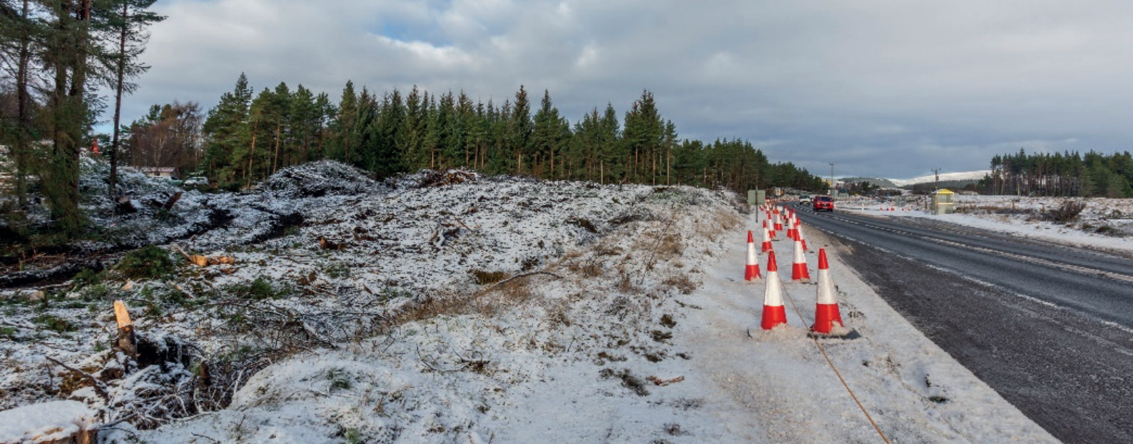
Image: Site clearance works alongside traffic management
